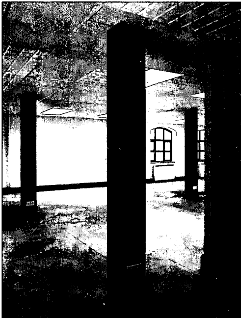
Figure 7.10 Board protection (Vicuclad, courtesy of Promat Ltd)
